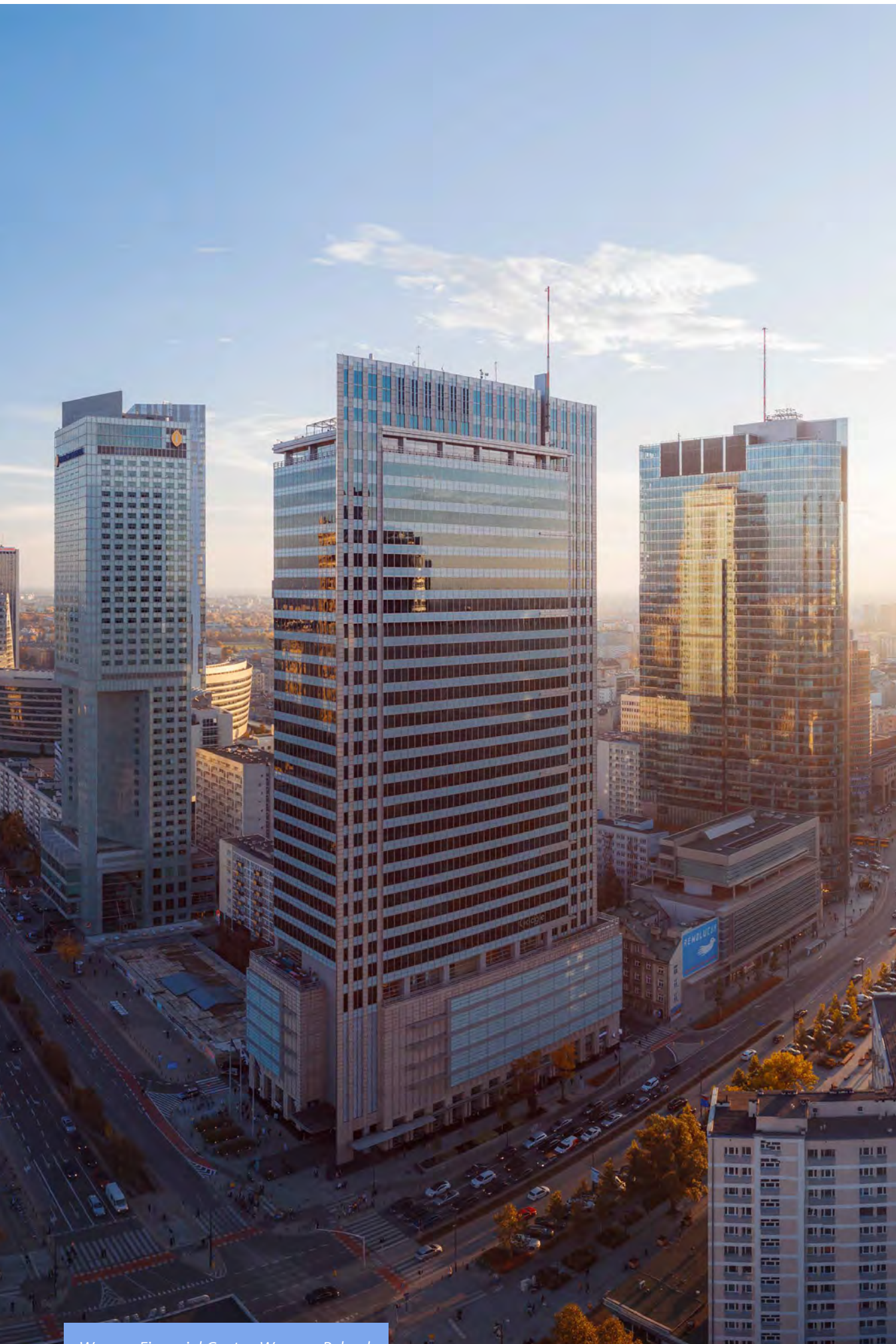
Warsaw Financial Center, Warsaw, Poland
